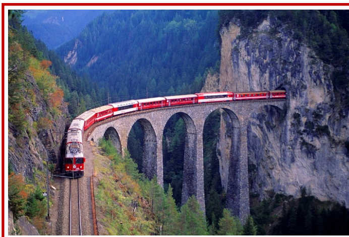
The most iconic feature of the Albula line is the Landwasser Viaduct between Filisur and Tiefencastel. Constructed of limestone, it has a span of 136 metres and is 65m high.
